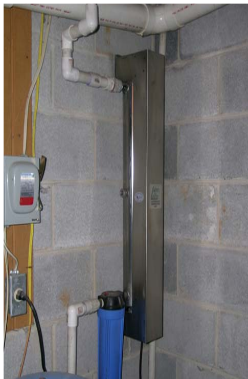
Figure 2. A typical UV light installation with a small canister sediment filter (bottom) ahead of the UV light unit.
